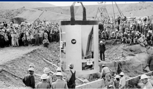
1957 Priest Rapids Dam First-Pour
